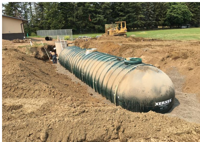
Pea gravel back-fill is used directly adjacent to the tank.
