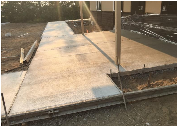
Yesterday's concrete pour turned out very nice.
