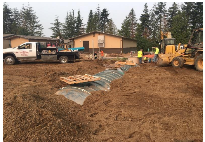
Tank back-fill is nearly complete.
