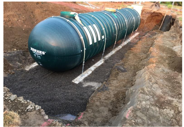
Septic tank installation included concrete tie-downs and straps.
